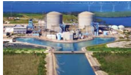
Nuclear power plant on Hutchinson Island, FL
